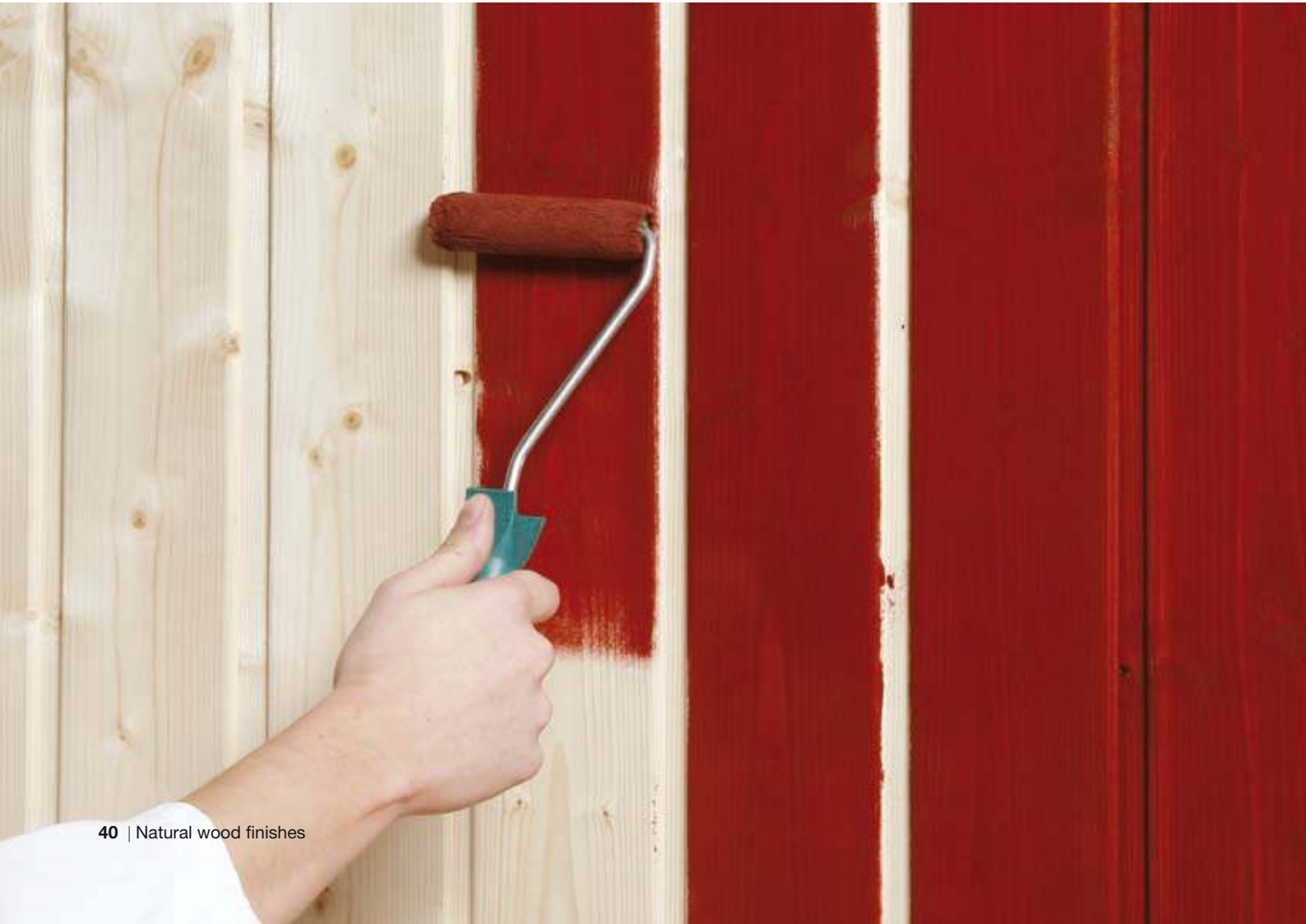
Application of Osmo Country Colour with the Osmo Roller and Brush Set
