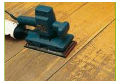
To renovate a floor, the lacquered surface must first be sanded down.
