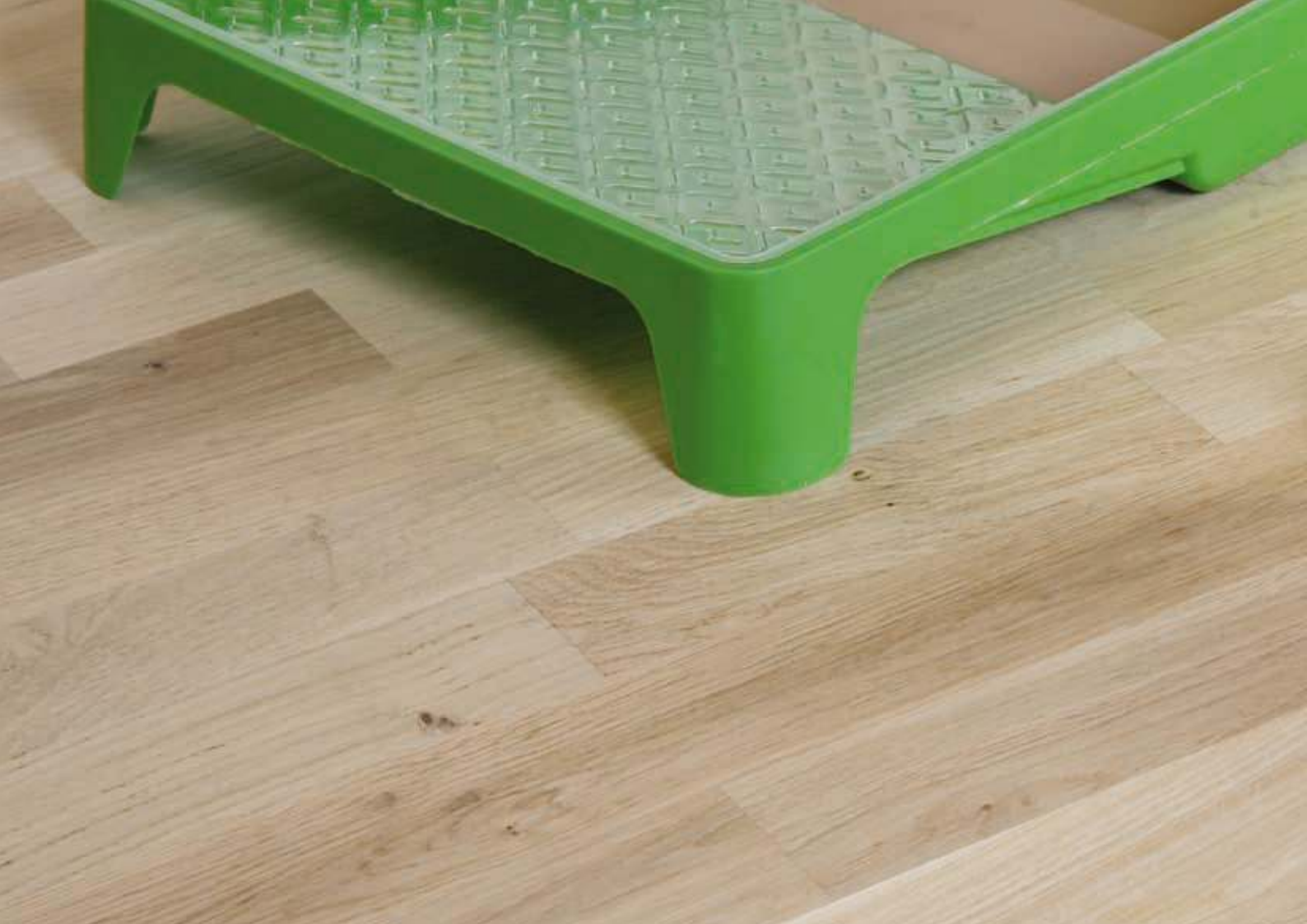
Applying Osmo Polyx®-Oil with the Osmo Floor Brush
